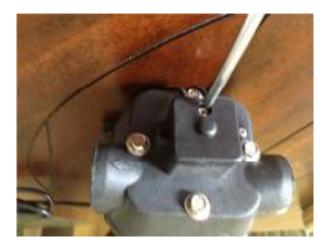
3. Disconnect the two wires.
