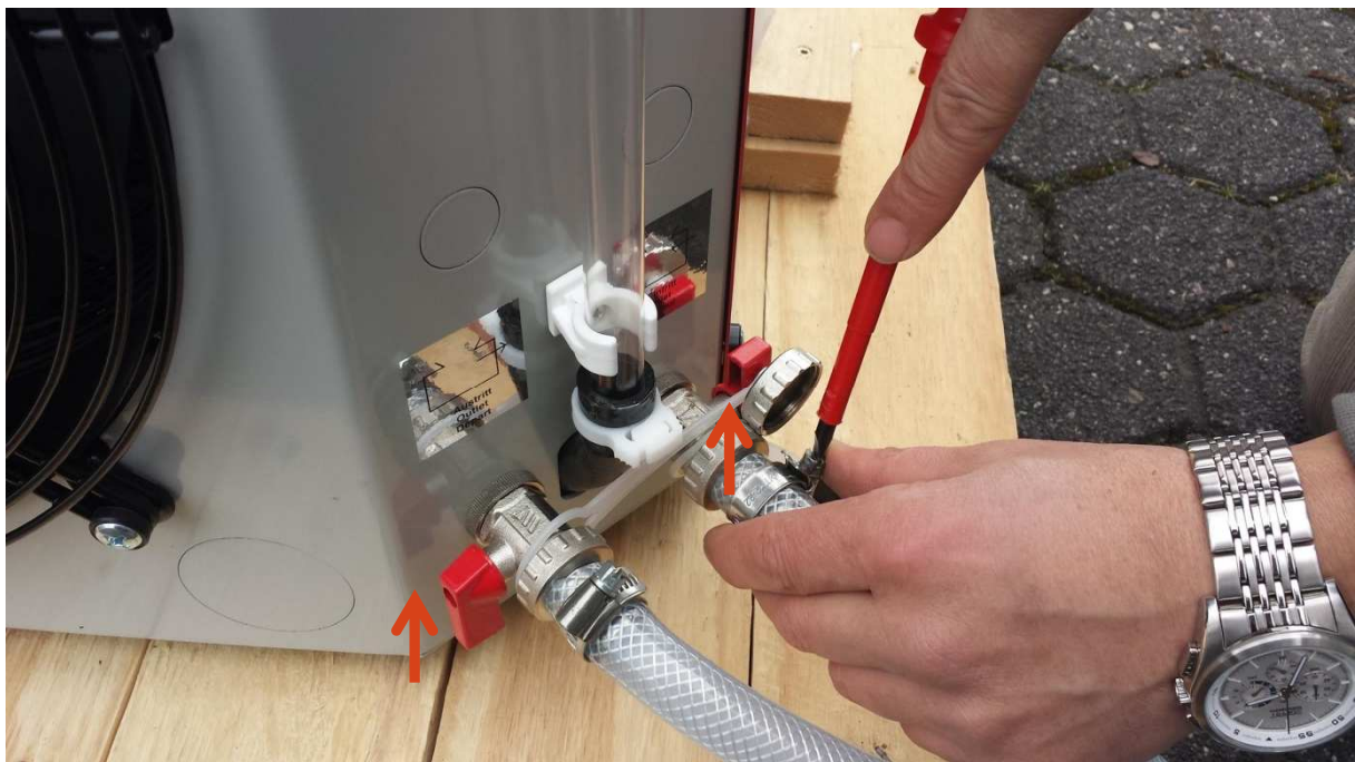
Pic. 7 + 8: Connection of the systems water pipes/hoses to the chiller. At this point the valves are closed and pointing upwards (see arrow direction).
