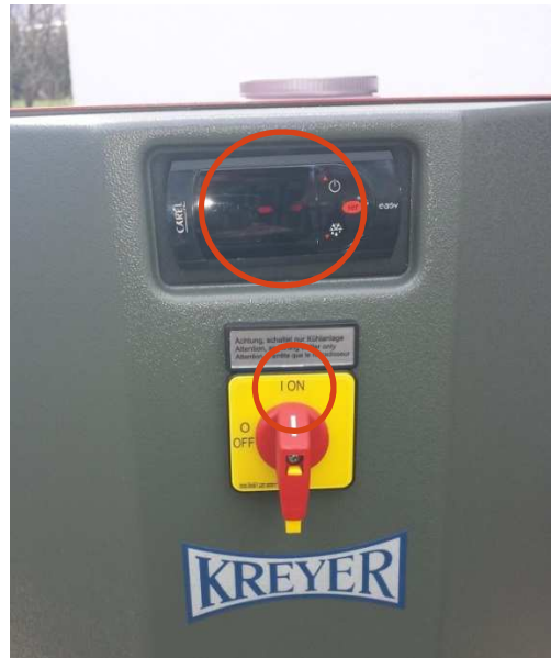
Pic. 13 + 14: Switching on the unit by turning the main switch to ON (dashed line appears in the display)
