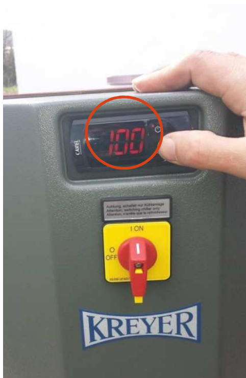
Pic.15 (left): Adjusting the Set-Temperature ( this picture is in Celsius degrees, in the next page and in the official manual you will find how to change your unit to show F° Fahrenheit degrees)
