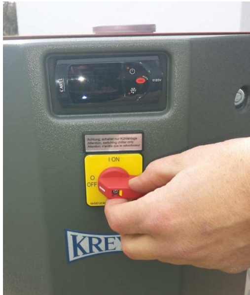
Pic. 13 + 14: Switching on the unit by turning the main switch to ON (dashed line appears in the display)
